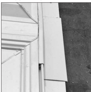
FIGURE 2 – ONE SIDE OF A STACKED UNIT COMPLETED. SILL WOULD BE SIMILAR
